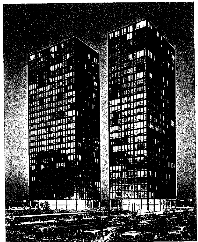
23.10 Mies van der Rohe, Lake Shore Drive Apartments, Chicago, 1951.
